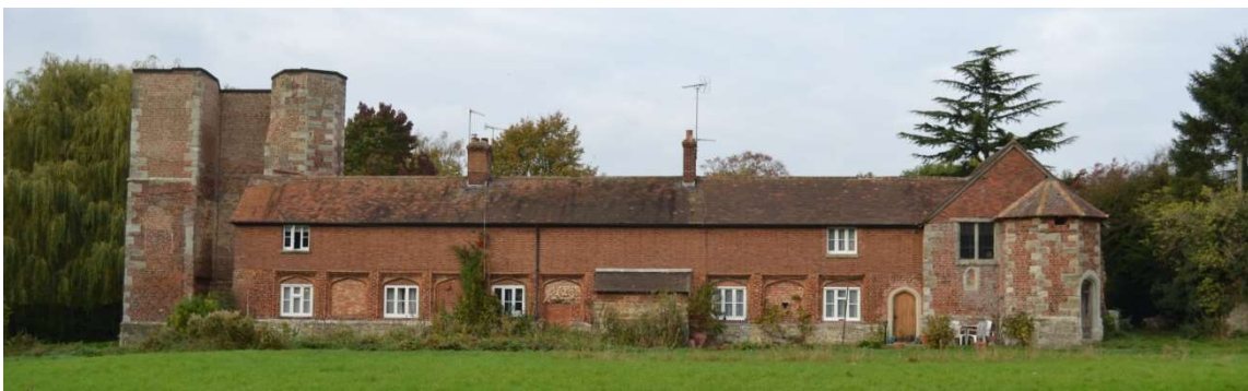
Figure 3: The view from the South after the first phase of repairs in 2016
